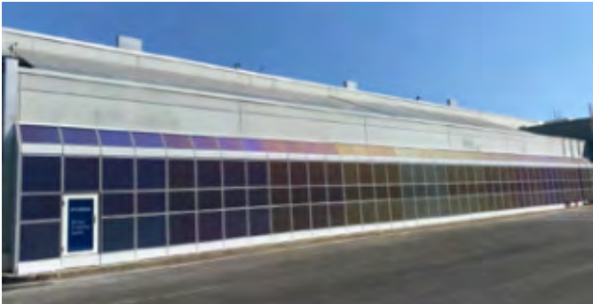
BIPV System at Eumseong Plant
